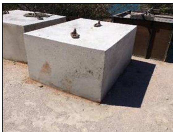
Five ton concrete mooring block used for longlines in Big Bay, Saldanha Bay
