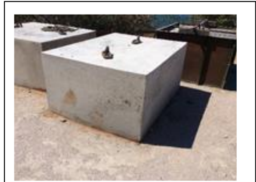
Figure 8: Five ton concrete mooring block used for longlines in Big Bay, Saldanha Bay.
