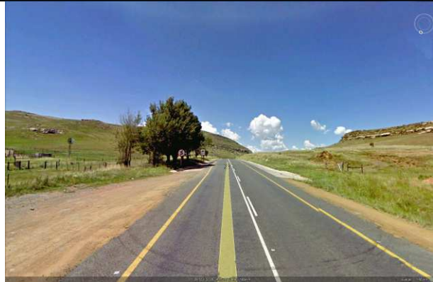
10. End of works at top of pass looking south.
