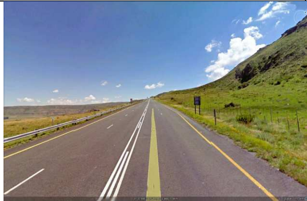
8. The double-lane section of road at mid-pass at km 63.8.
