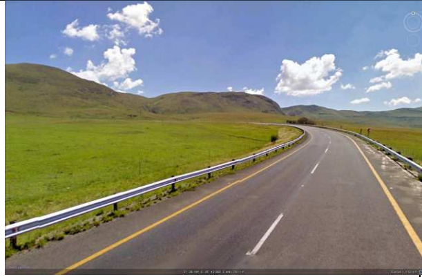
6. Start of the big bend in the road at km 61.3.
