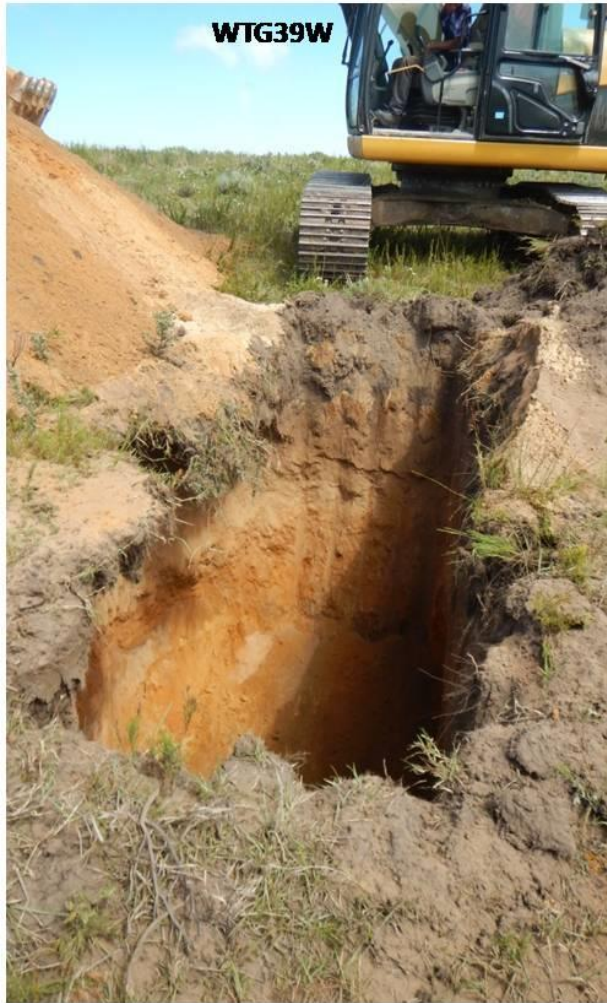
Plate 17. Geotechnical test pits at WTG39, 40 and 41W. Excavations are between 4 and 5 m deep. No archaeological traces or anthropogenic layers were seen.
