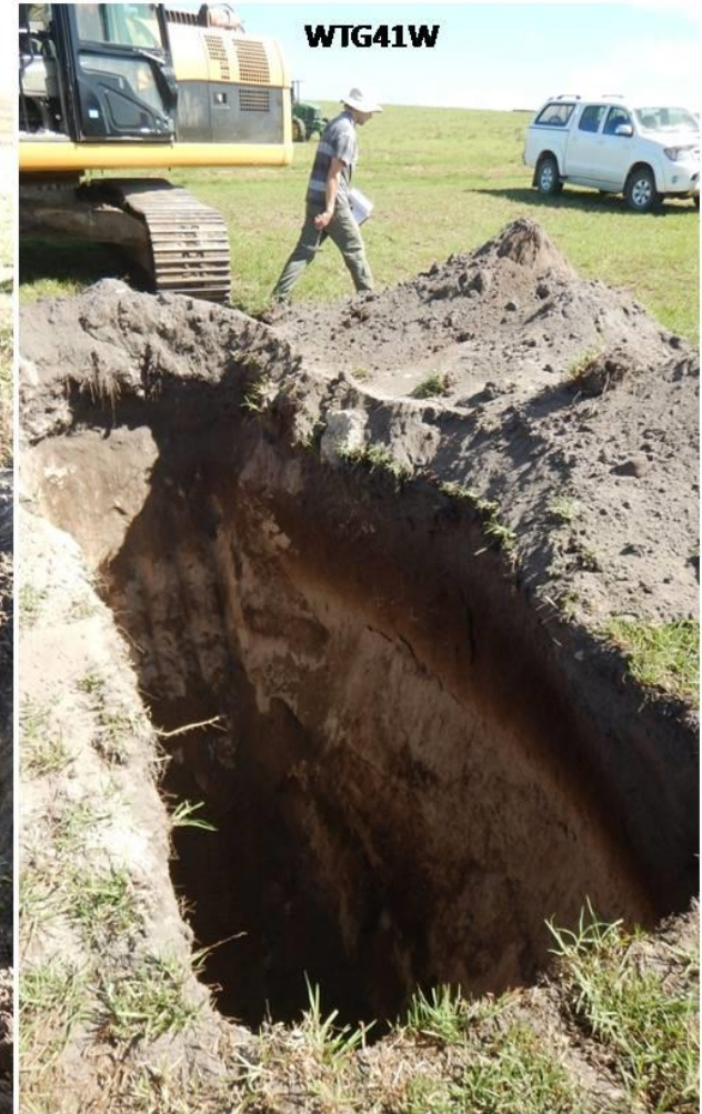
Plate 17. Geotechnical test pits at WTG39, 40 and 41W. Excavations are between 4 and 5 m deep. No archaeological traces or anthropogenic layers were seen.
