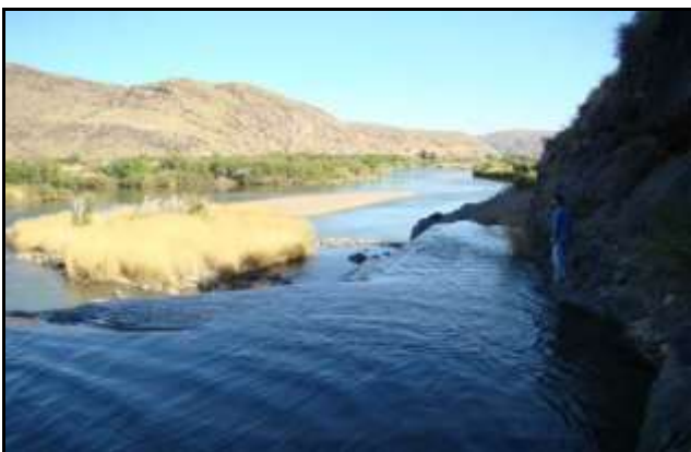
Figure 3: View of the small cliff at the north-eastern end of the weir.
