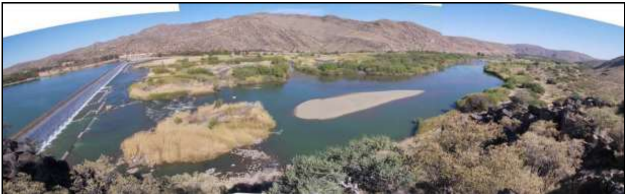
Figure 2: View from above the Boegoeberg weir showing the character of the river valley at this point. The photograph is taken from the top of the small cliff below which the power station would be built.
