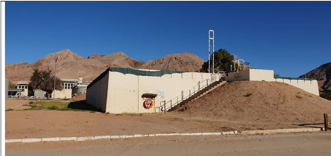
Plate 7: Existing Water Treatment Plant
