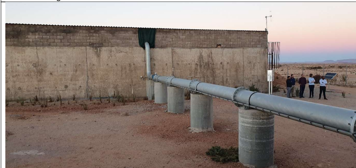
Plate 9: Existing Horseshoe Reservoir 2
