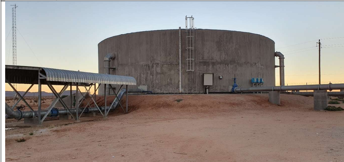
Plate 8: Existing Horseshoe Reservoir 1
