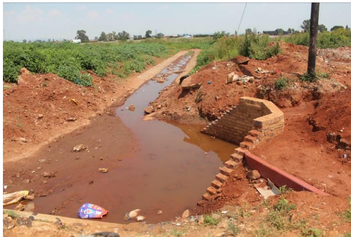
Figure 5: Storm water drainage line on the study site.
