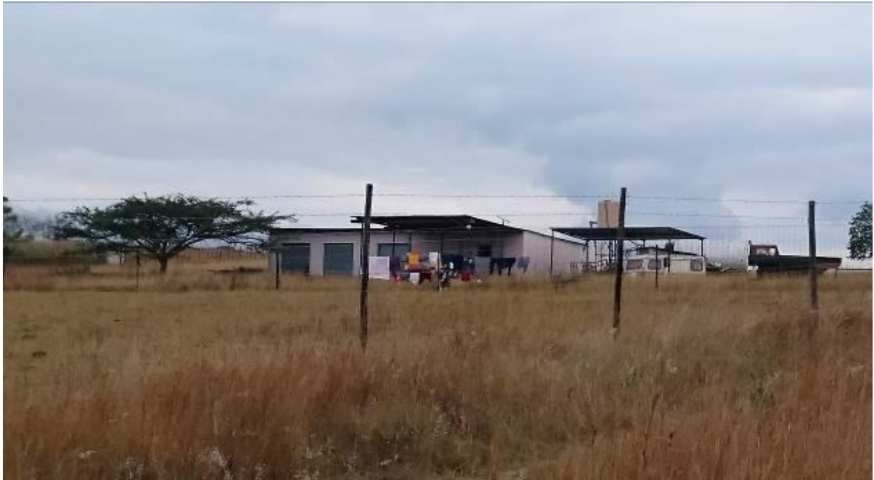
Plate 9: Dwelling in corridor AE
