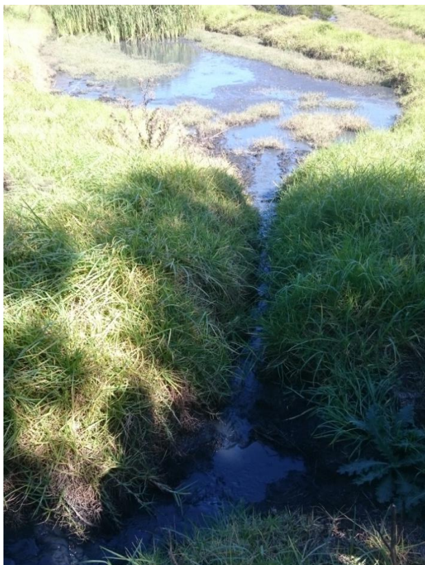
Photo 8 Existing stormwater channels diverting stormwater flow around secondary evaporation ponds
