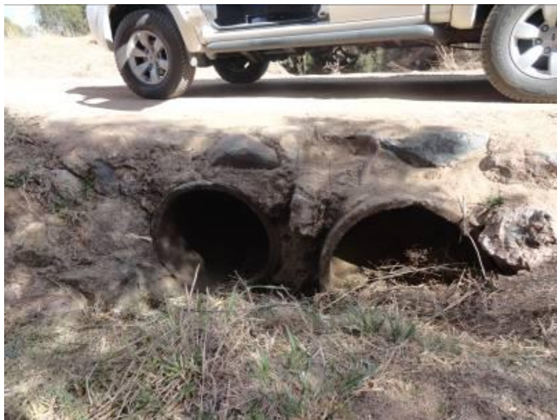
Figure 9, Low level culvert crossing.
