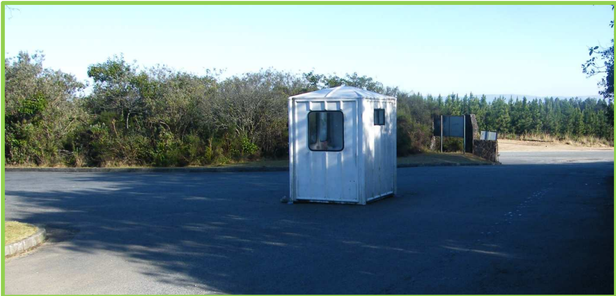
Figure 7: Entrance and Security Shelter.
