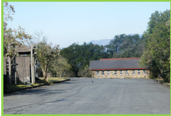
Current Ablution Facilities
