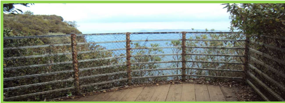
Railings at a viewing platform at God's window.
