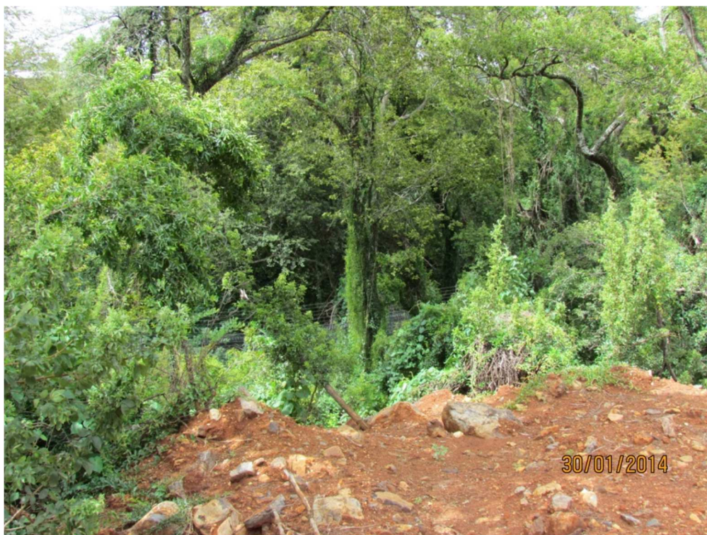
Figure 6: Encroachment of infilling into the riparian zone of the Sesmyslspruit and confinement of the 1:100-year floodline
