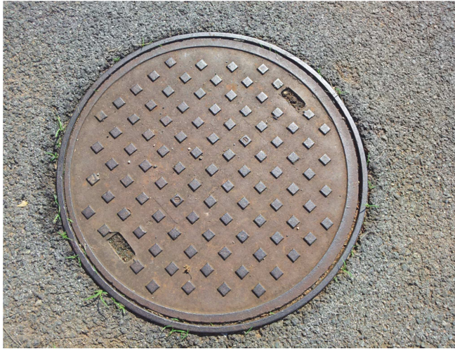
Plate4: BH02: Capital Park Primary School
