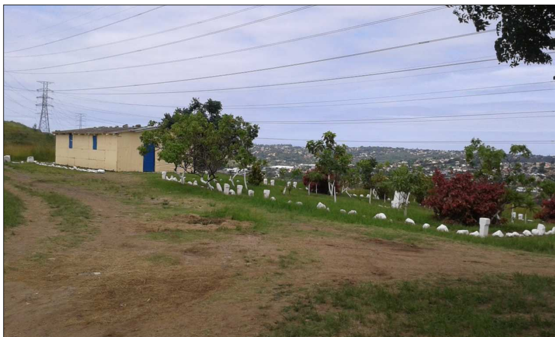
Figure 18: General view of the church with the rectangular building on the left and the area demarcated with white stones evident on the right.
