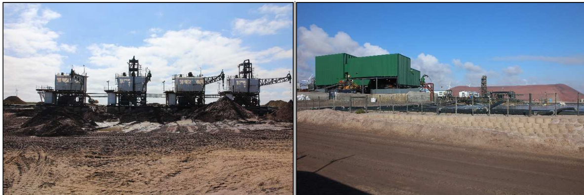
Figure 1: The PBCs (left) and the SCP and process water dams (right)
