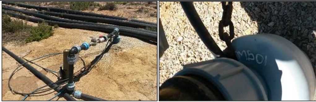
Figure 36: Borehole TMB01 – unable to measure water level and no longer in use
