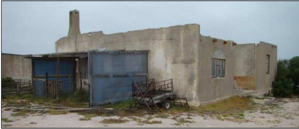
Figure 78: The “Police Station” on Geelwal Karoo 262
