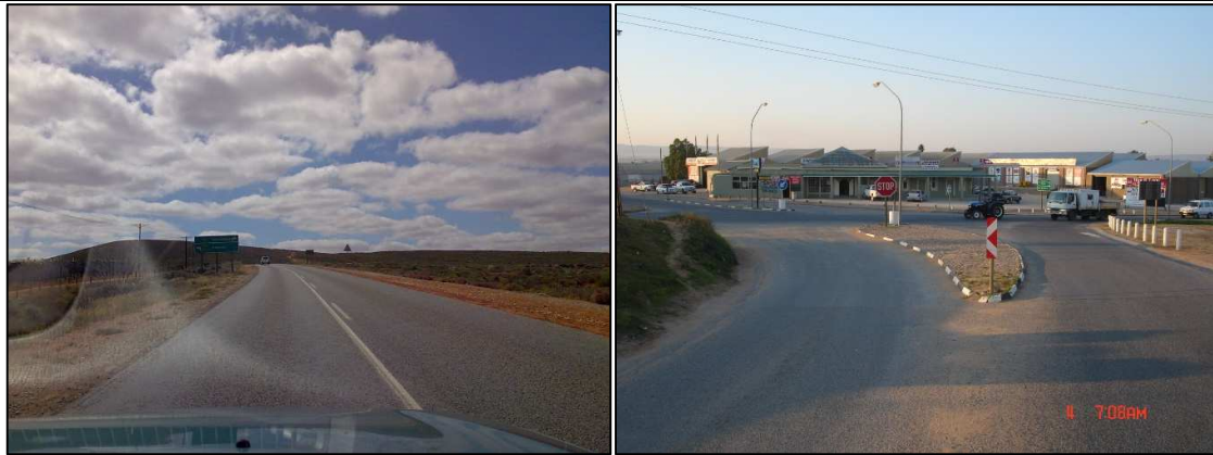
Figure 87: Northbound view along the R362 (MR548) towards the R27 in Vredendal (left) and southbound view along R362 (MR552) towards the R27 in Vredendal (right)
