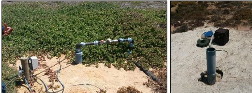
Figure 37: Borehole TMB04 – unable to measure water level and no longer in use (left) and Borehole TPB01 – dry to 30 m (right)
