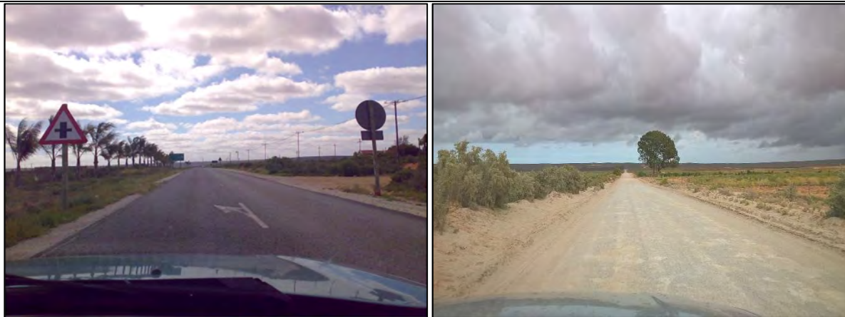
Figure 99: Northbound view along the R363 (MR547) towards Koekenaap (left) and westbound view along the DR2225 from Koekenaap (right)
