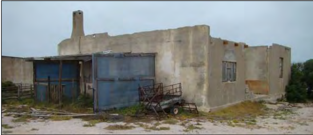
Figure 89: The “Police Station” on Farm Geelwal Karoo 262
