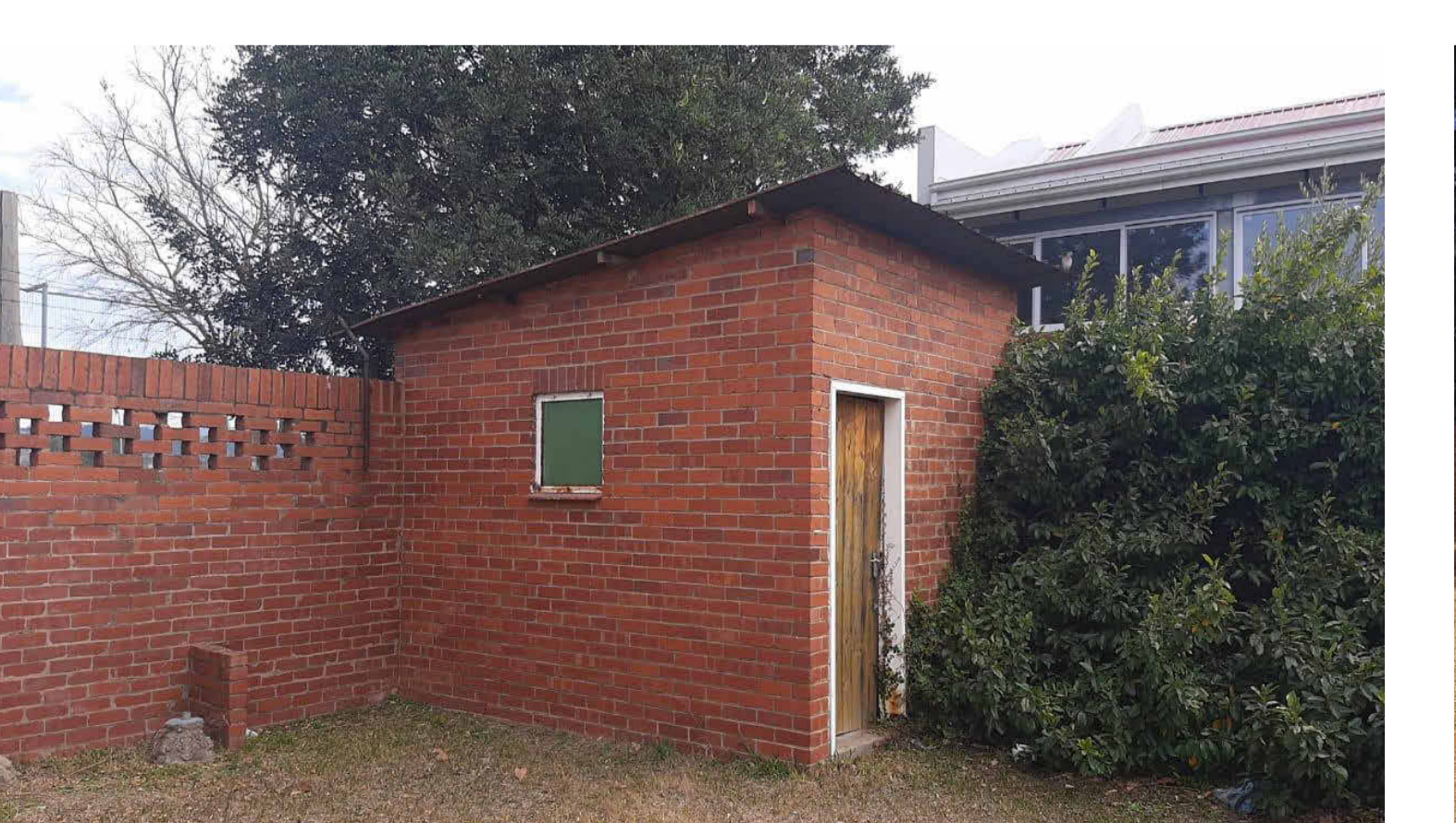
Photo of Existing Buildings #9
