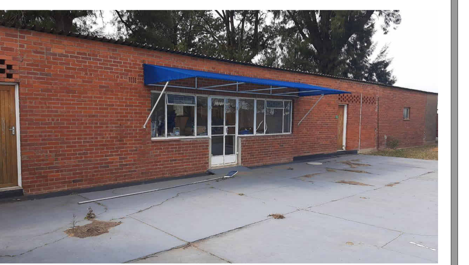
Photo of Existing Buildings #5
