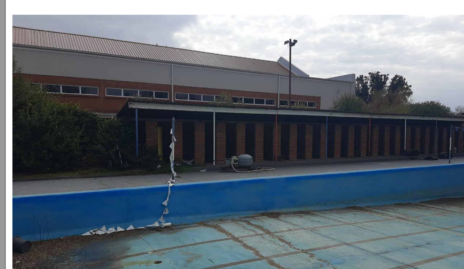
Photo of Existing Buildings #6
