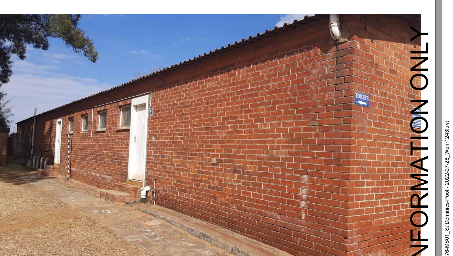
Photo of Existing Buildings #10
