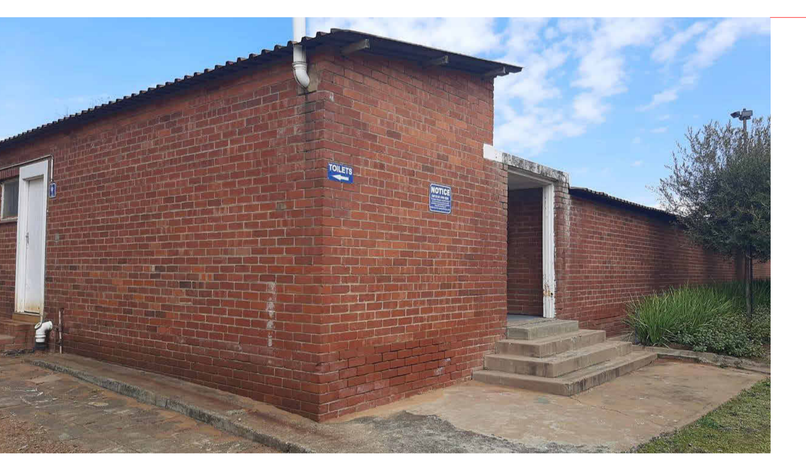
Photo of Existing Buildings #4
