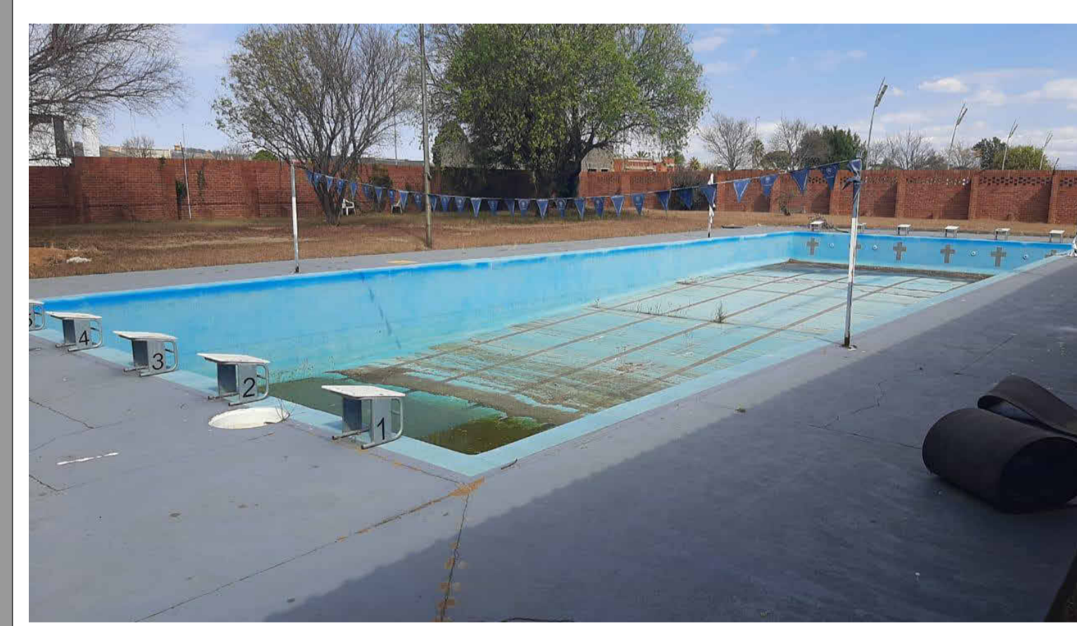
Photo of Existing Buildings #1
