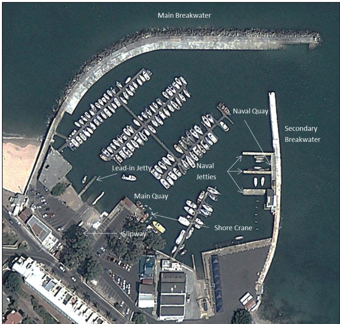
Figure 2-3: Structures at Gordon's Bay Harbour
