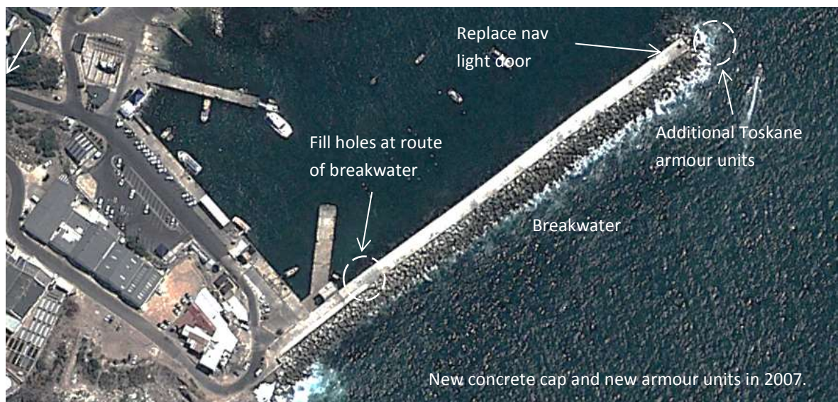
Figure 2-3: Main Breakwater Structure
