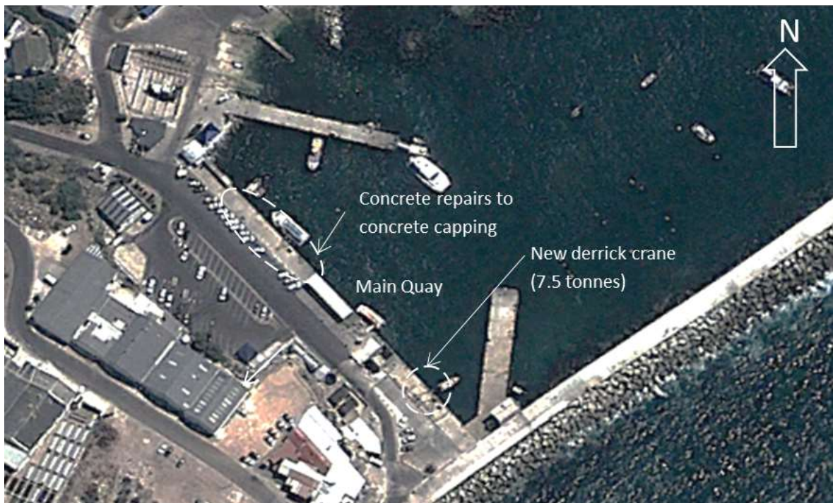
Figure 2-4: Main Quay Structure
