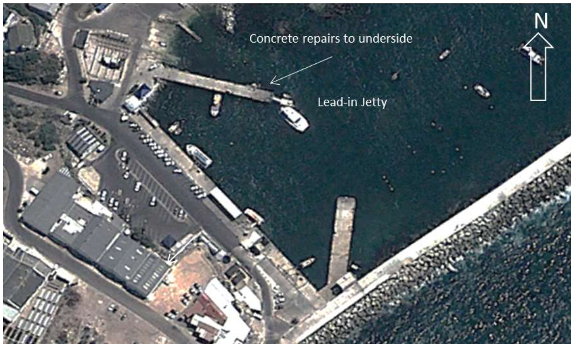
Figure 2-5: Lead in Jetty Structure
