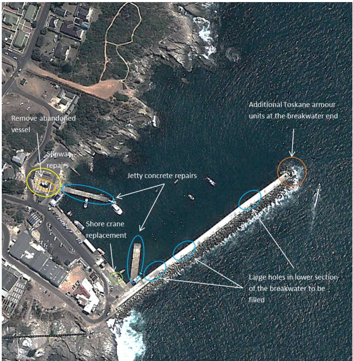
Figure 2-2: Work required in Hermanus Harbour
