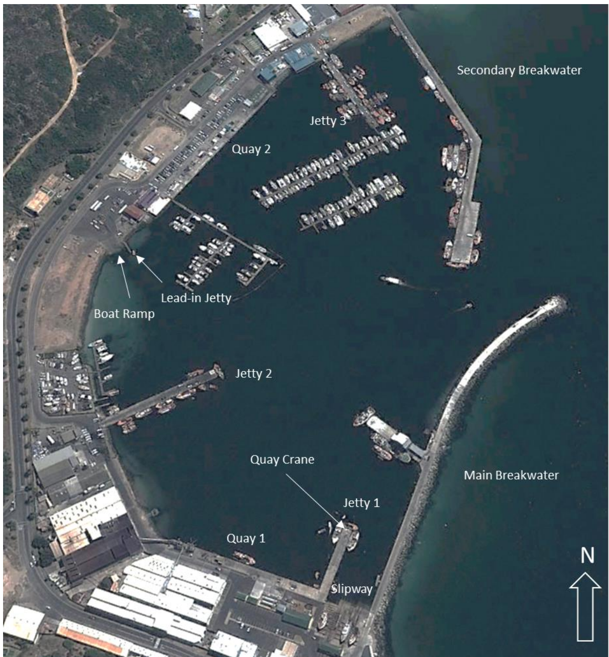
Figure 2-1: Hout Bay Marine Structures
