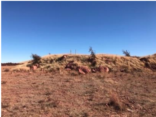
Figure 21: Soil and rock dumping within the eastern proposed soil stockpile and parkup area (facing west).
