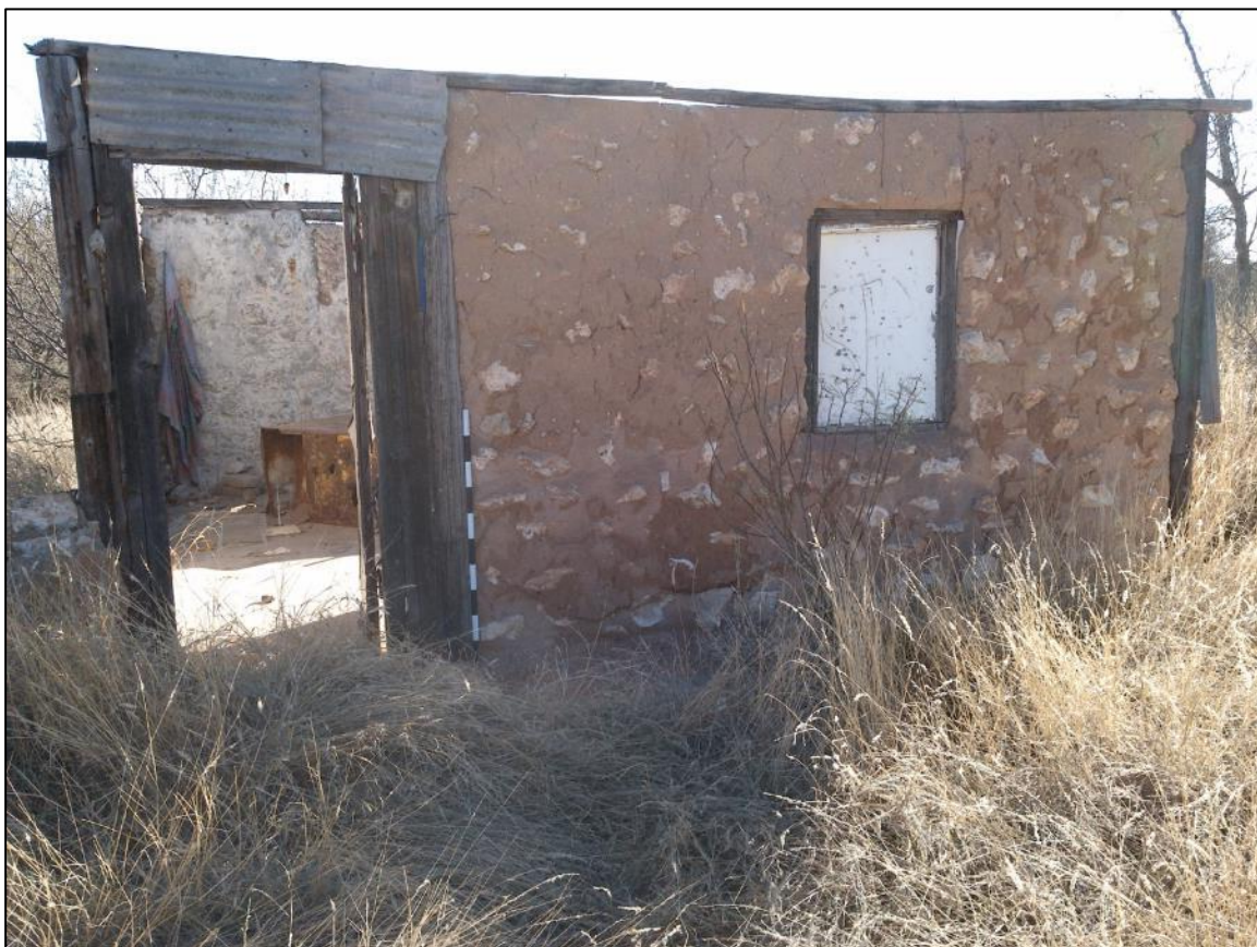
Figure 55 – View of the structure at site KLIP-003.
