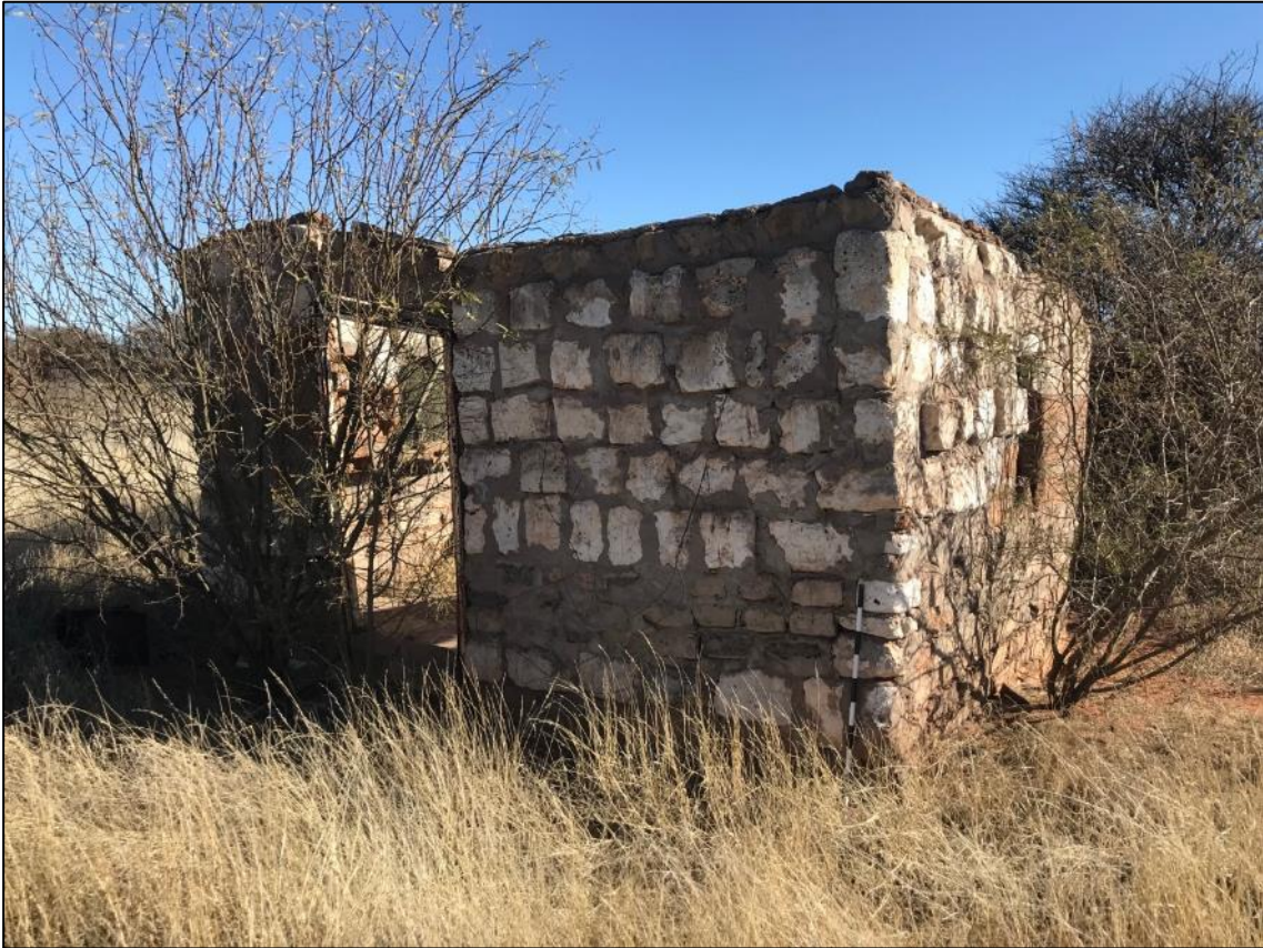
Figure 48 - View of the structure at site KLIP-001. The scale is in 10cm increments.
