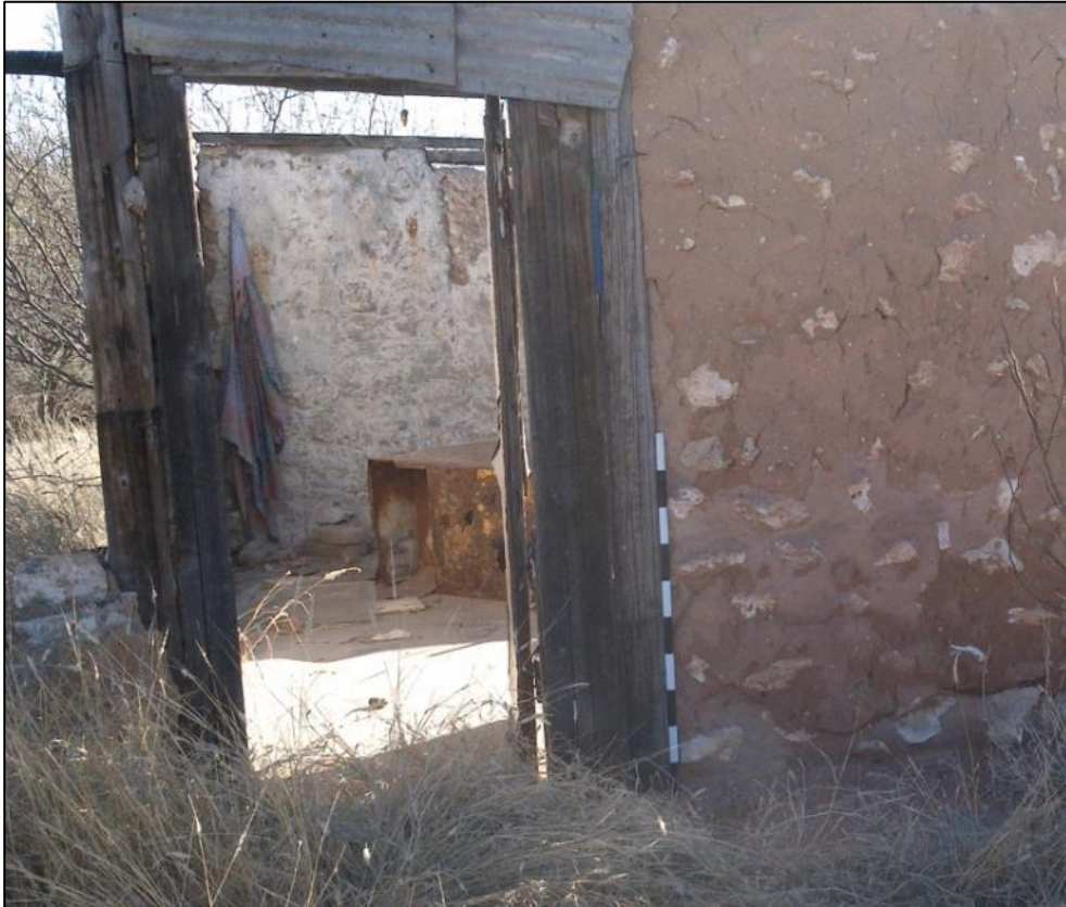
Figure 56 – Closer view of the door and interior of structure at KLIP-003.
