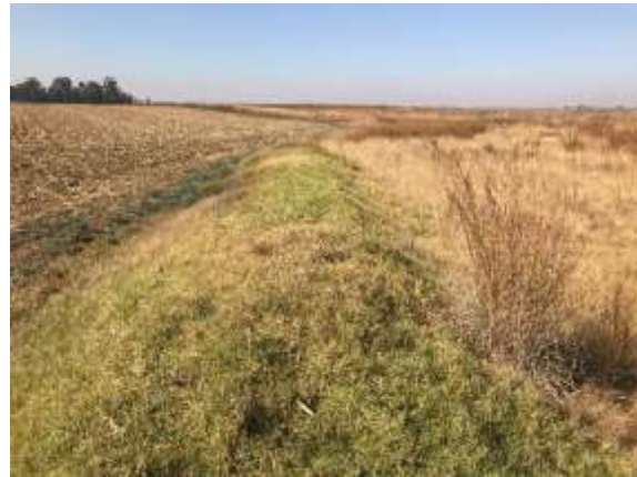
Photo 12: Earth berms are commonplace within the project area that have been historically established to increase the cultivation potential of the agricultural sector.
