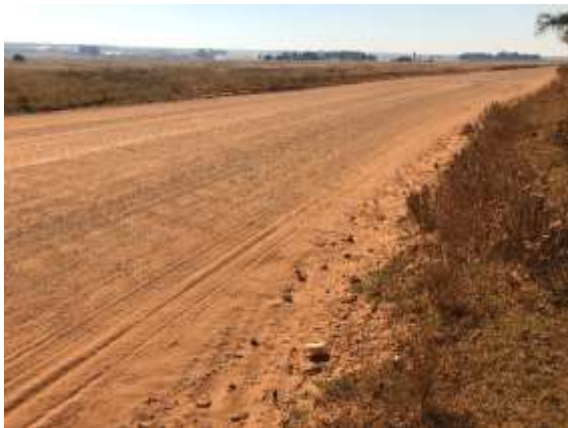
Photo 7: A section of the existing gravel road to be rehabilitated.
