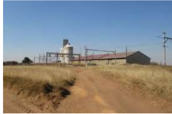
Photo 6: Grain silos situated along the D684.
