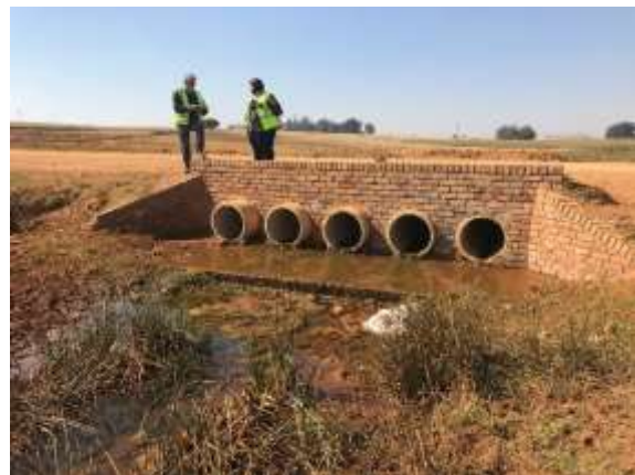
Photo 20: The bridge design of the main watercourse, showing the series of side-by-side culvert pipes.
