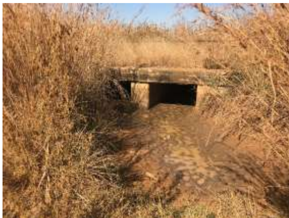
Photo 13: Existing bridge/culverts. This allows surface water drainage beneath the existing railway.
