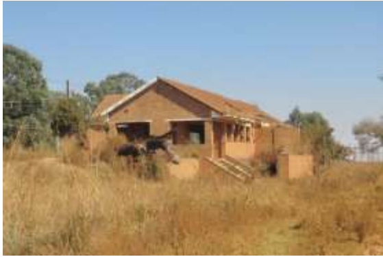
Photo 5: Vandalised Arnot Railway Station situated along the D684
