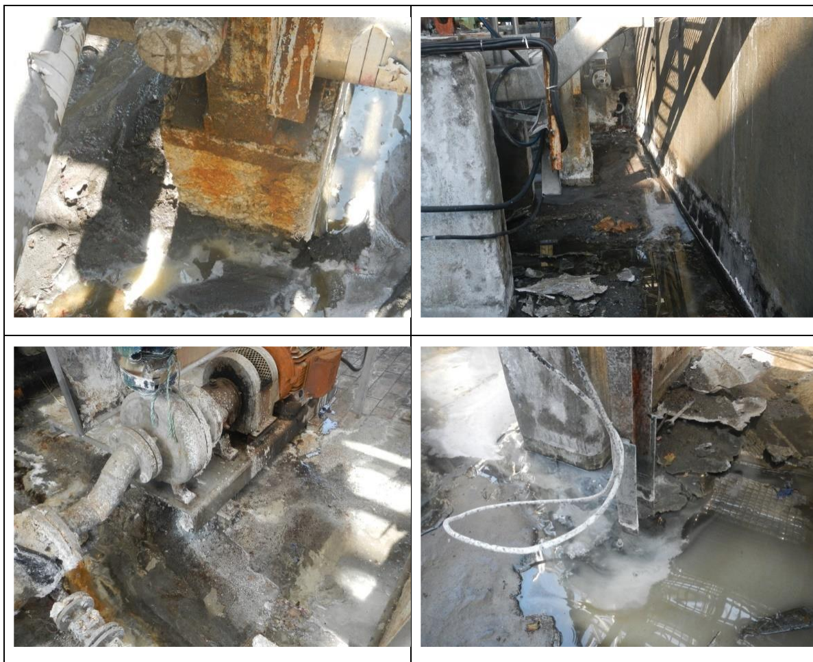
Figure 1-2: Situation at the Current Bulk chemical storage facility
