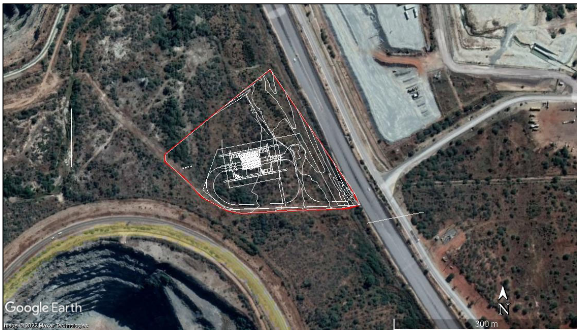
Figure 19 - The construction of the proposed development footprint area enclosed by the red polygon is not expected to have any significant impact on the old mining remains.
