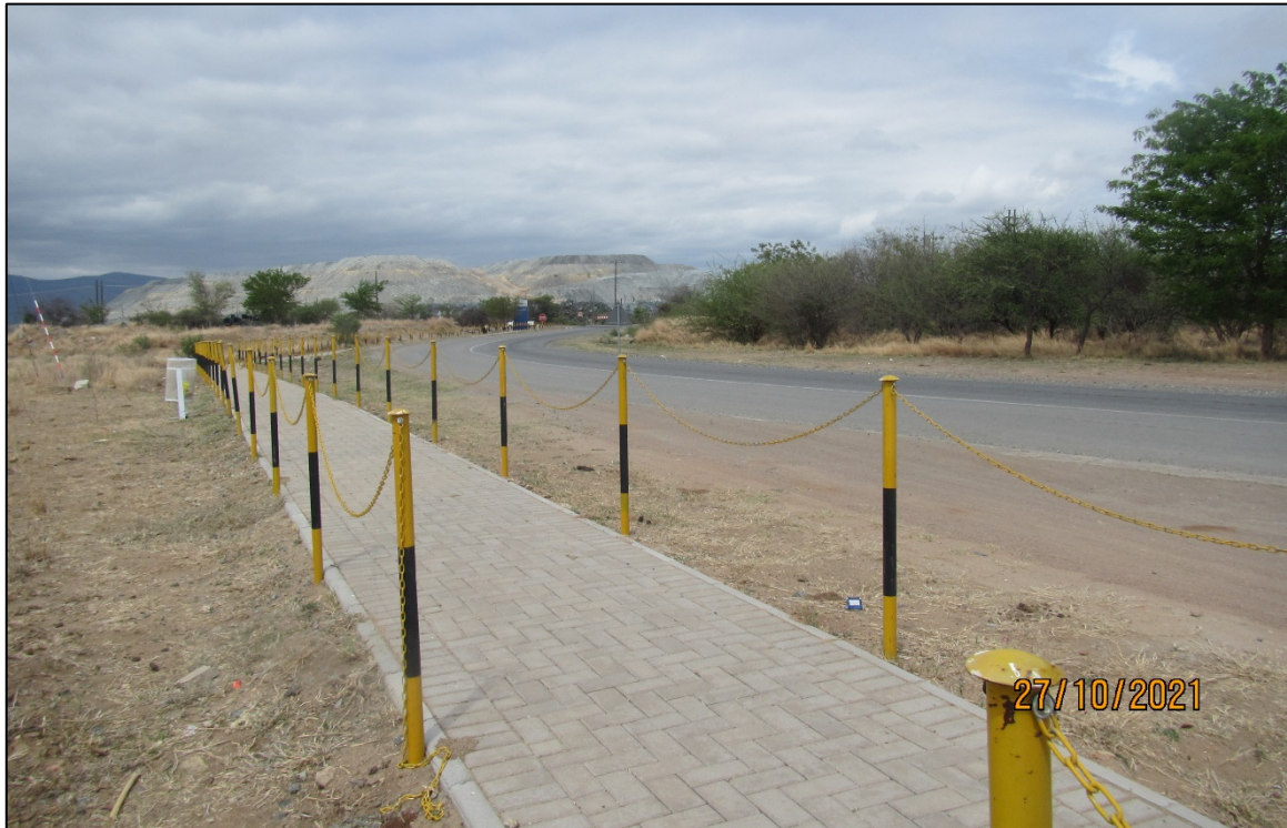
Figure 10 - View of the access road to the Mogalakwena North Concentrator. This road is located to the north of the project area.
