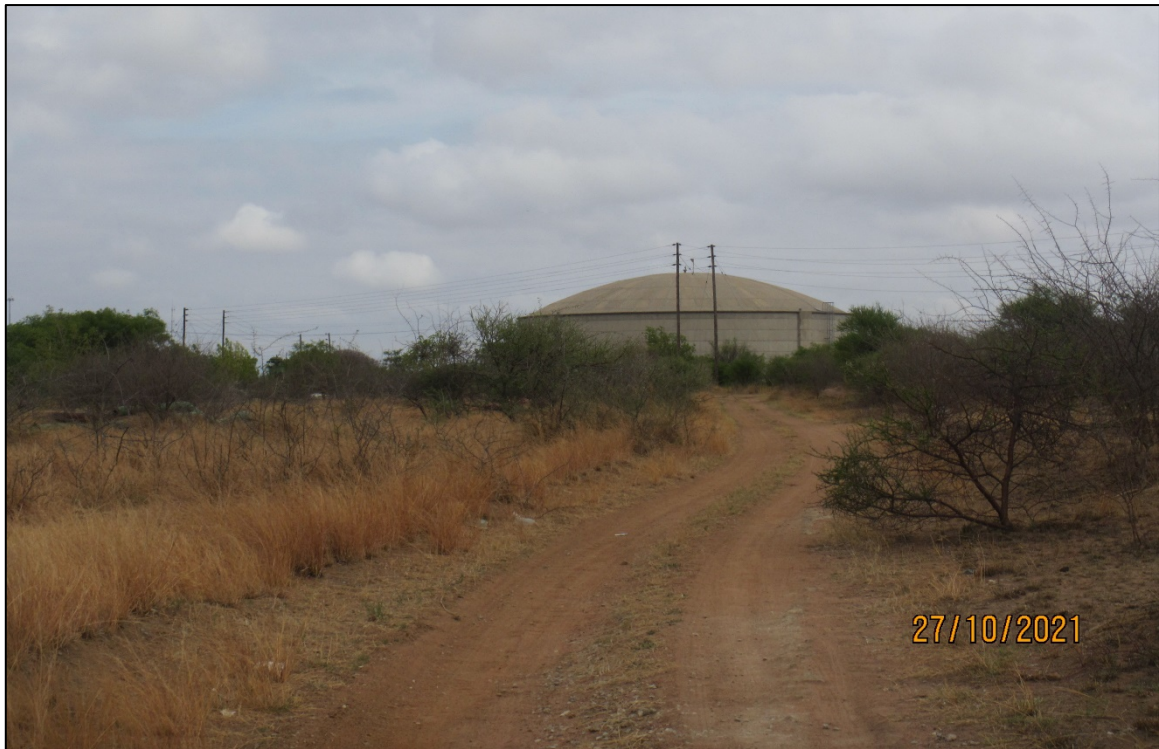
Figure 8 - A water reservoir and treatment plant are located to the north of the project area.
