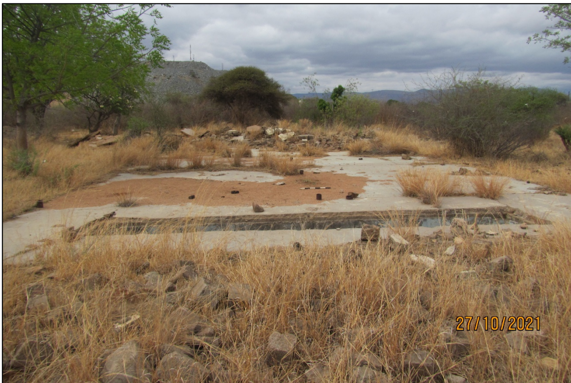
Figure 24 - View of the remains of a concrete floor of a larger building. A vehicle inspection or grease pit can be seen within the structure. This supports the information provided by a community member who indicated that a mechanical workshop was located here.
