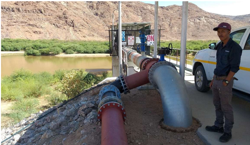
Figure 5: Existing water extraction point for the bulk water pipeline (January 2020)
