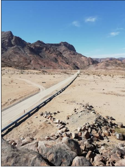
Figure 7. General site conditions.
