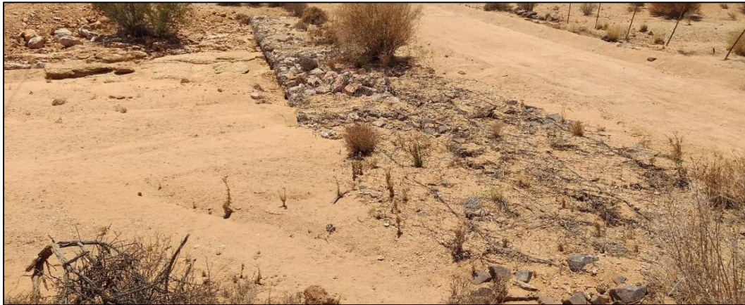
Figure 15: Ephemeral river crossing the dirt road (January 2020)
