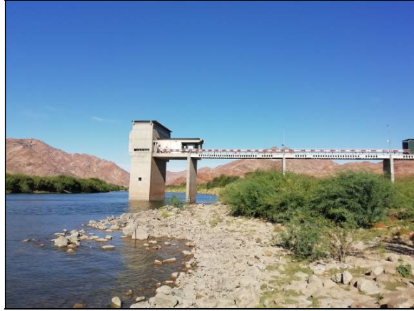
Figure 8. Abstraction tower at the Orange River
