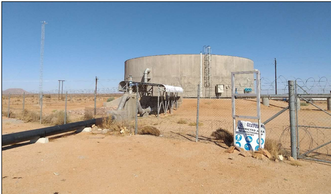
The horseshoe reservoir, the endpoint of the pipeline (January 2020)
