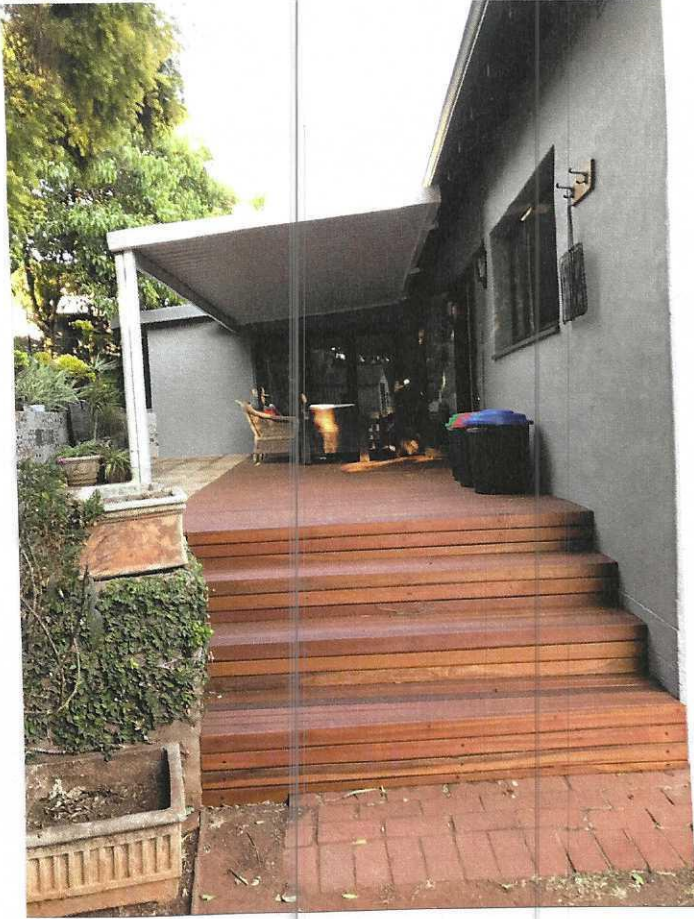
North Elevation of patio area
