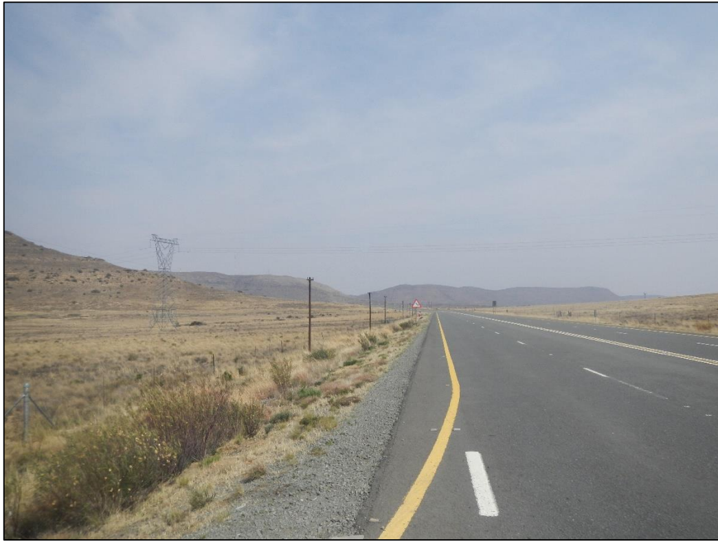
Figure 24: View of high voltage power lines traversing the N9 national route.
