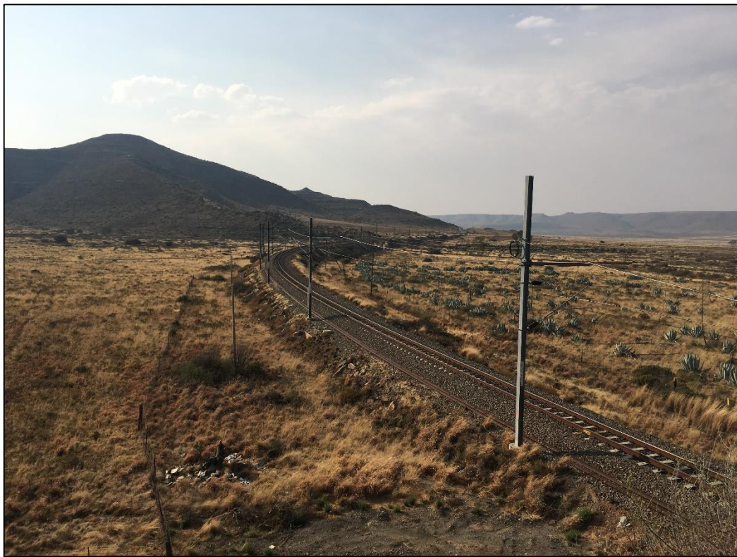
Figure 23: Railway infrastructure in the study area.
