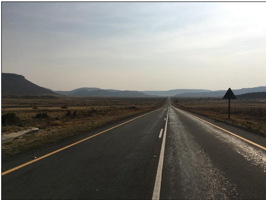
Figure 25: View of the N10 national route in the south-western sector of the study area.
