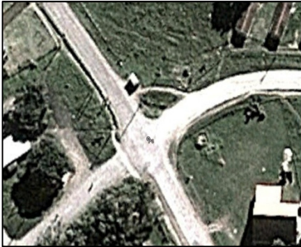
Figures 6.10: Aerial view of intersection
