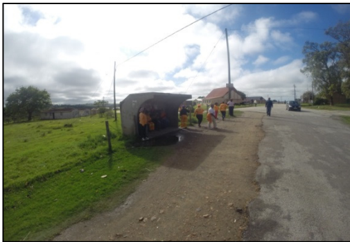
Figure 8.1: Public transport stop with shelter near the A Street/Khonza Street intersection
