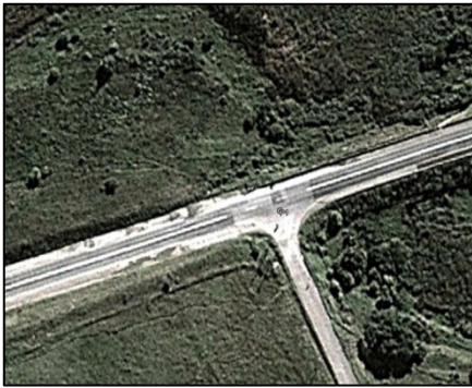
Figures 6.5: Aerial view of intersection
