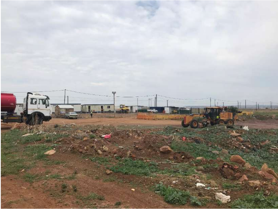
Figure 5: Road construction site camp on the western portion of the site.
