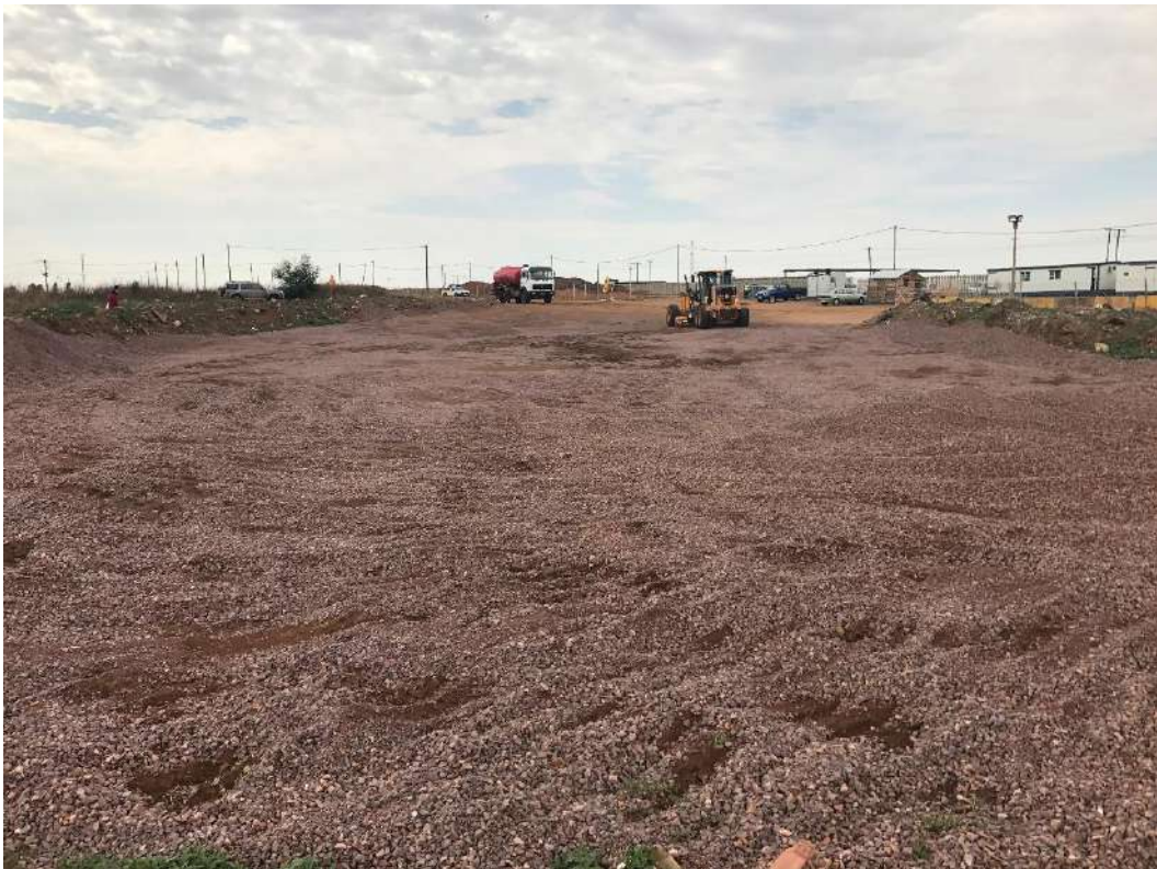
Figure 6: Stone stockpile for road construction.
