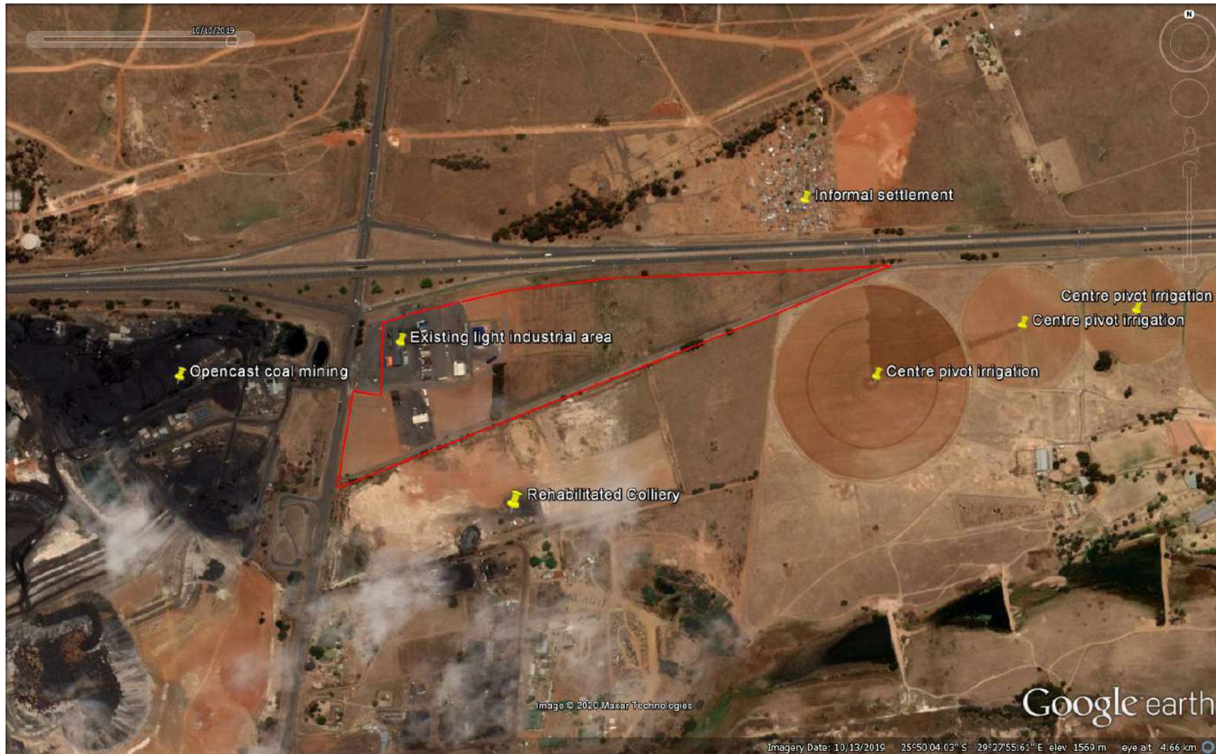
Figure 14 Recent aerial imagery showing the land uses and surrounding land uses of the project site
