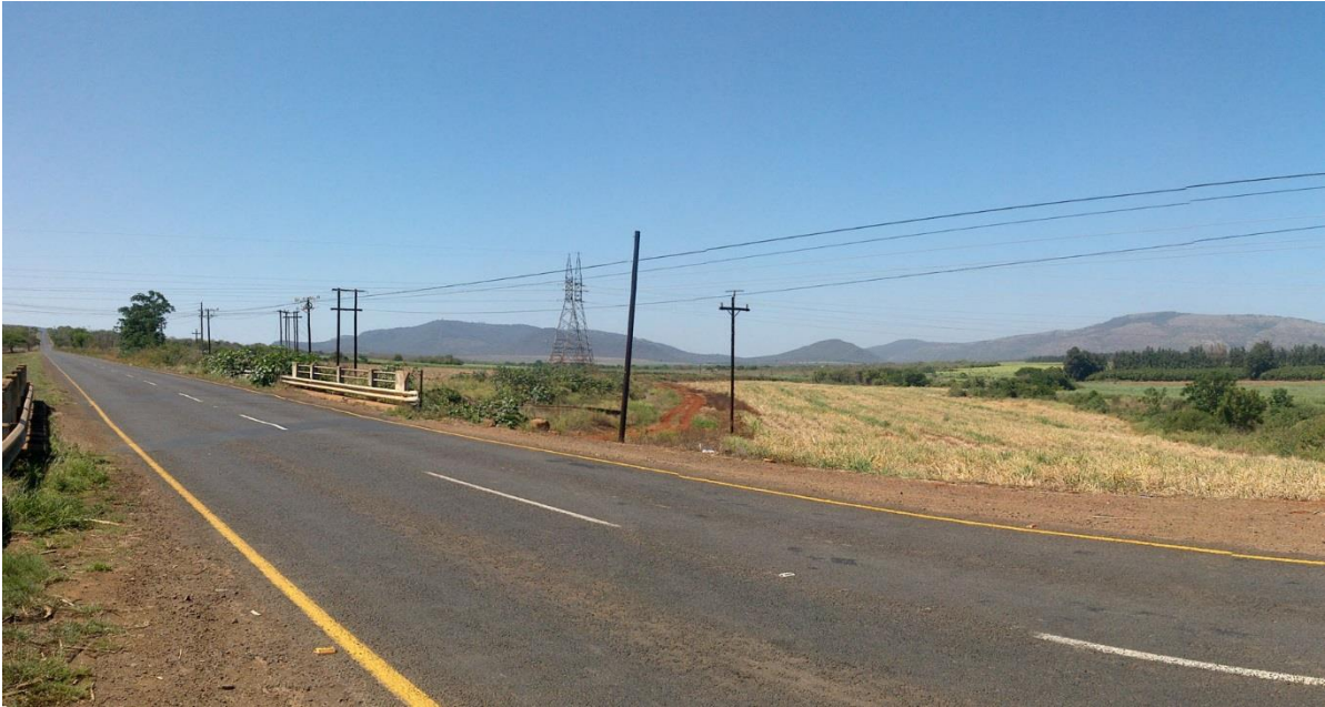
Figure 6-6: Disturbed landscape with existing powerline south of Pongola (Viewpoint E)
