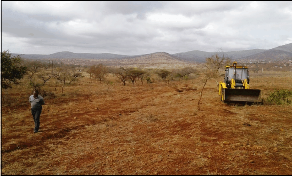
Plate 4: The western drainage line parallel to the western boundary.
