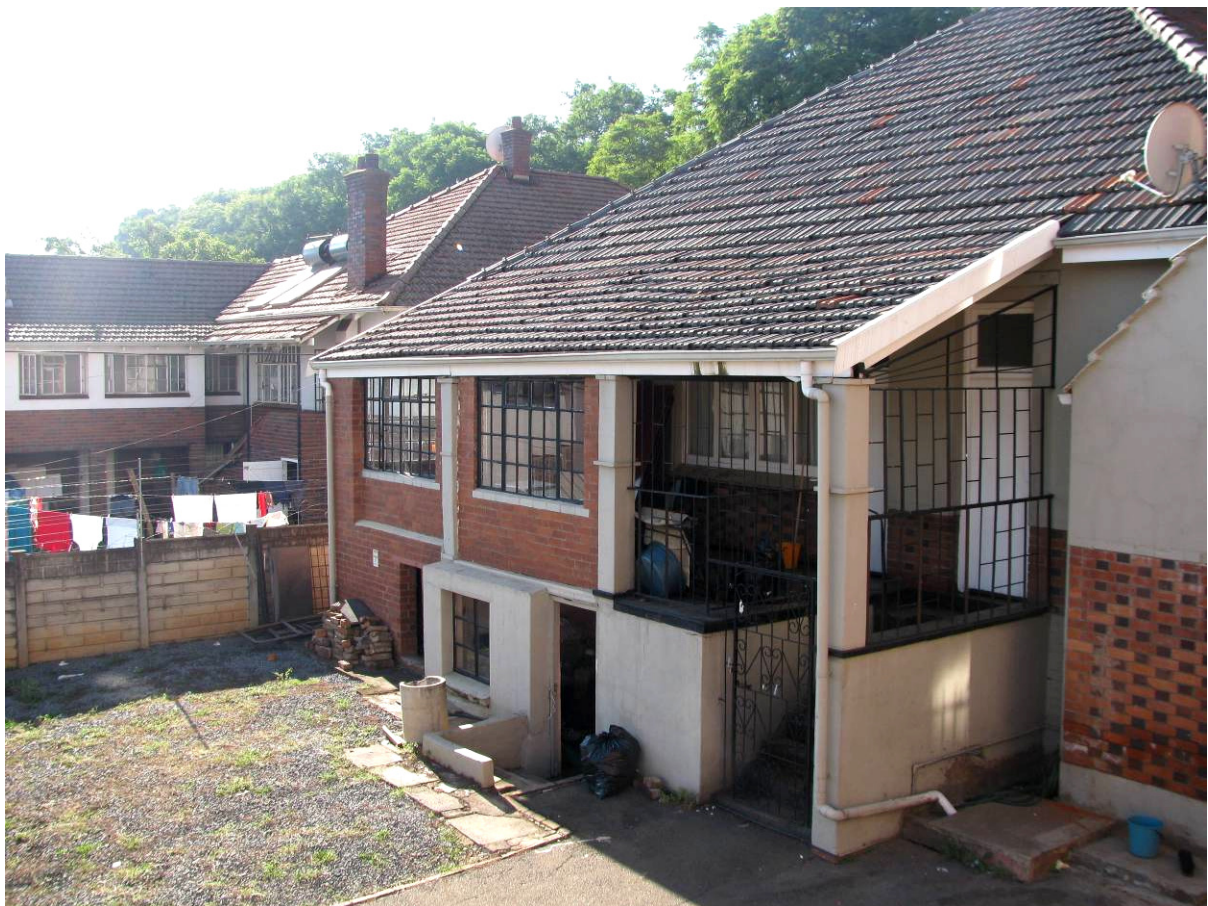
North West Elevation (back of house)
