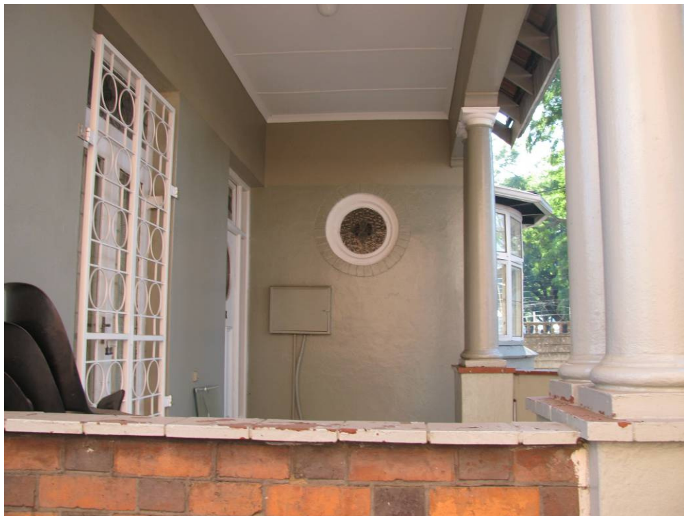
Veranda view, facing North East
