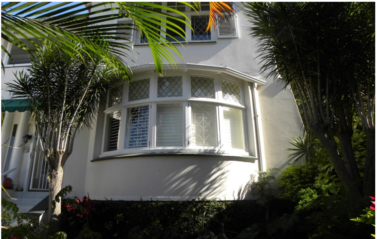
FRONT OF HOUSE SHOWING EX. BAY WINDOW
