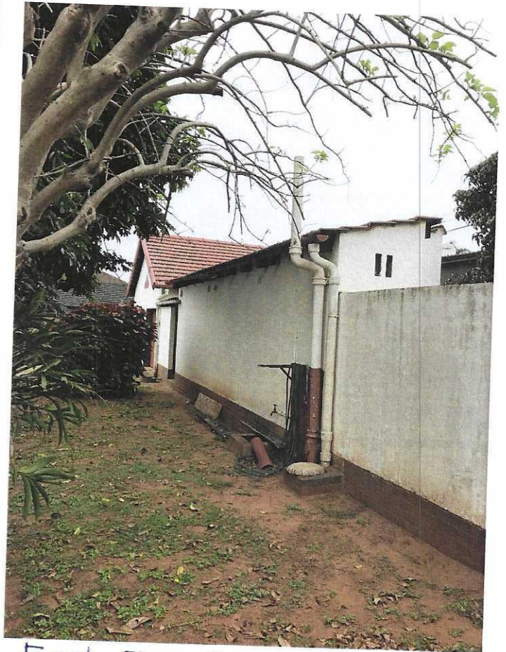
East Elevation - outbuilding
