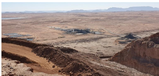
Figure 3. Gamsberg Mine Existing Infrastructure
