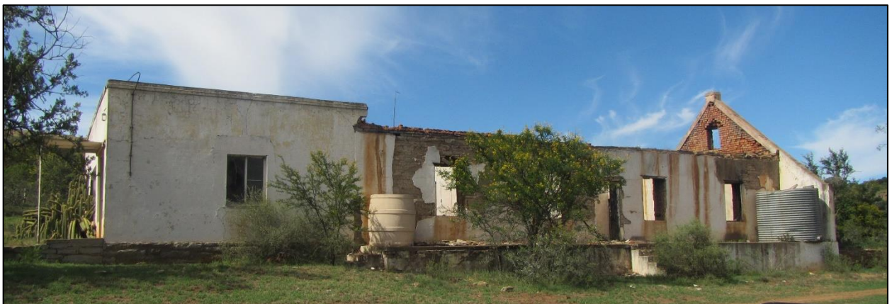
Figure 28: Ruined farm house at waypoint 1729. It likely dates to the mid-19 th century but has more recent additions to the east end (left side in this view) and rear.
