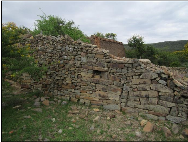
Figure 26: The other side of the stone wall visible in Figure 25.
