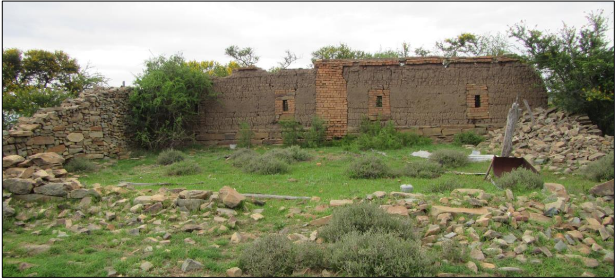
Figure 25: Ruin and stone kraal at waypoint 1710. The building has a stone foundation and a combination of sundried bricks (brown) and fired clay bricks (orange) in the walls.
