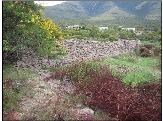
Figure 27: Another section of stone walling on the kraal at waypoint 1710.
