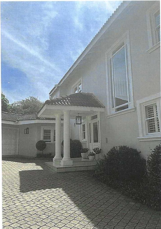
S.W. Elevation - Entrance Porch
