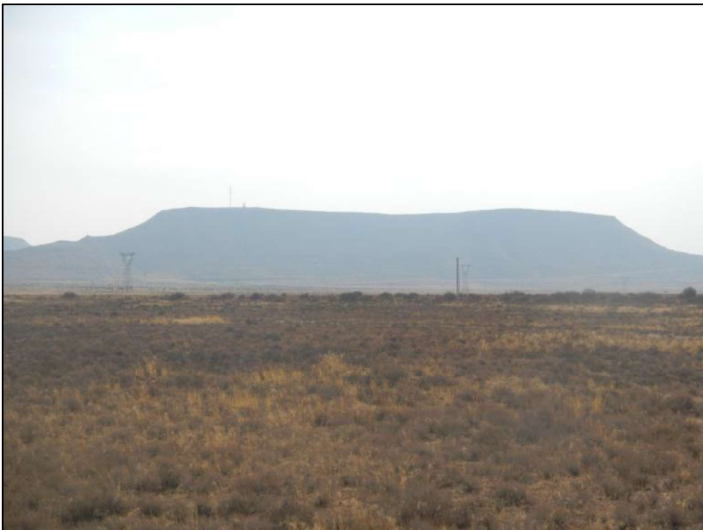
Figure 40: View of the existing power lines from VR 36.
