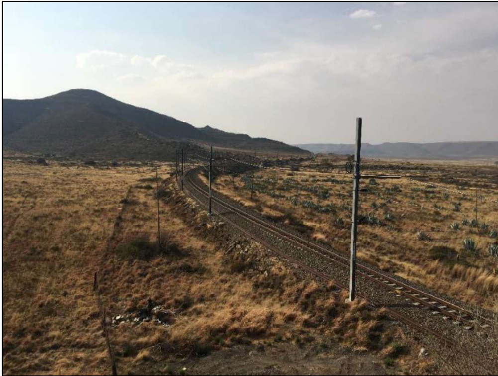
Figure 25: View of the railway line which traverses the study area in a north-south direction.
