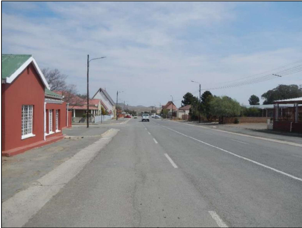
Figure 28: View from within the town of Noupoort showing the urban visual character.
