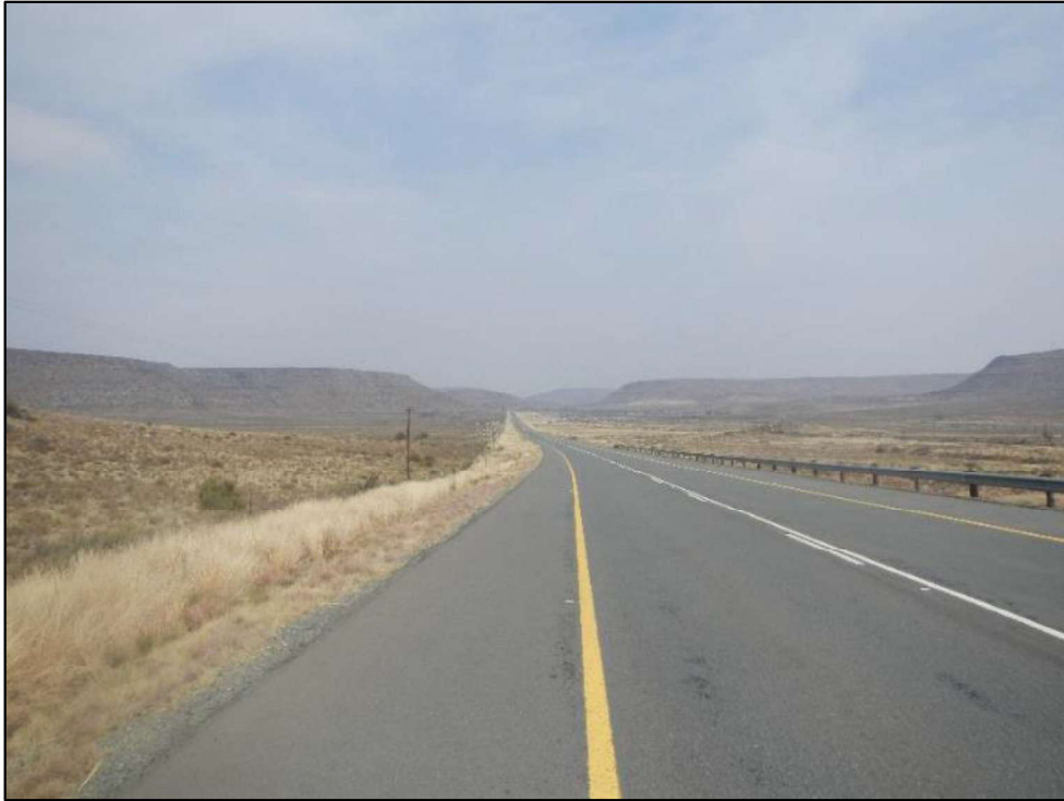
Figure 22: View of the N9 national route which traverses the study.
