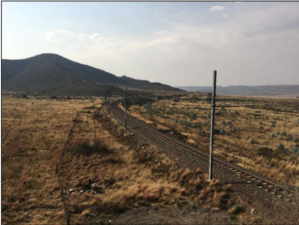
Figure 23: View of the railway line which traverses the study area in a north-south direction.
