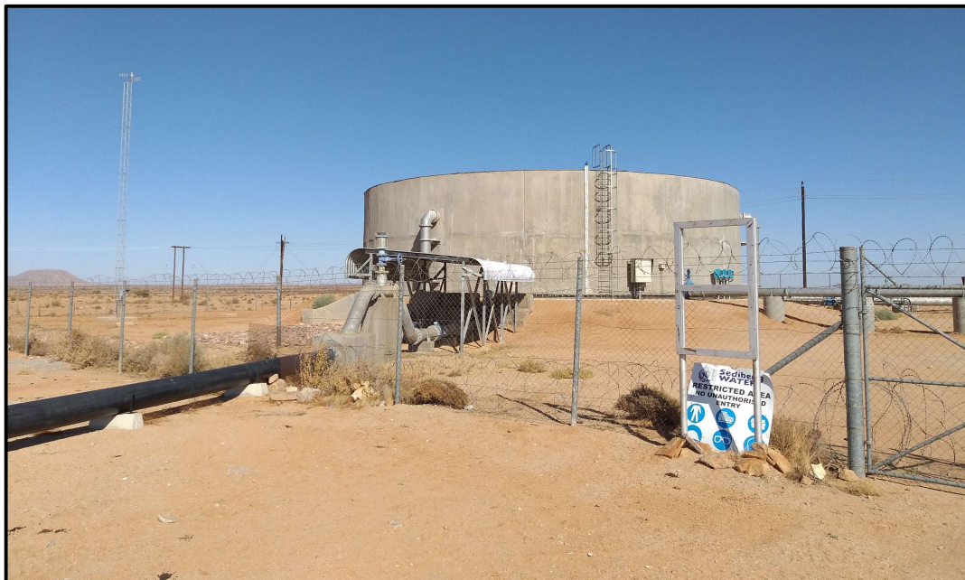
The horseshoe reservoir at the end of the project area (January 2020)
