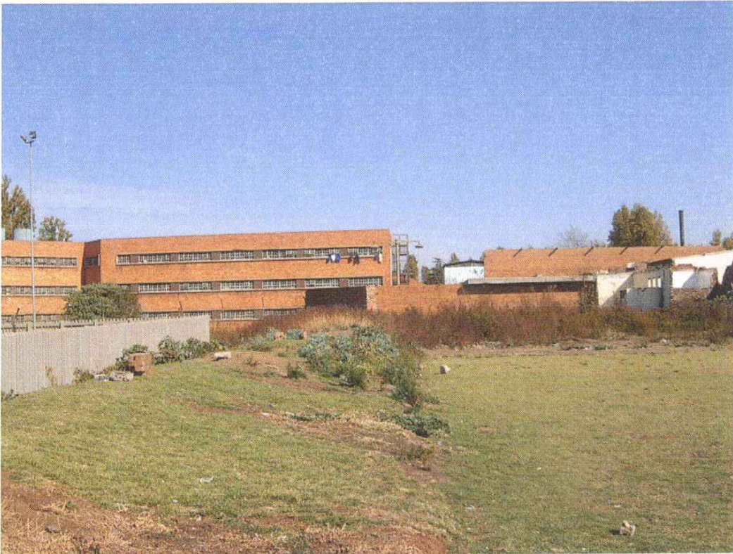
Photograph 6: View of Robert Strachan Hostel from Jan Hofmeyer Street on eastern boundary.
