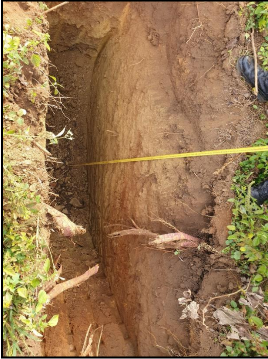
Plate 9: Indicative view of residual soils and deeply weathered shale rock at IP17
