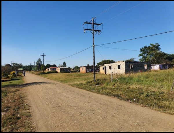
Plate 4: General view of route of bulk pipeline
