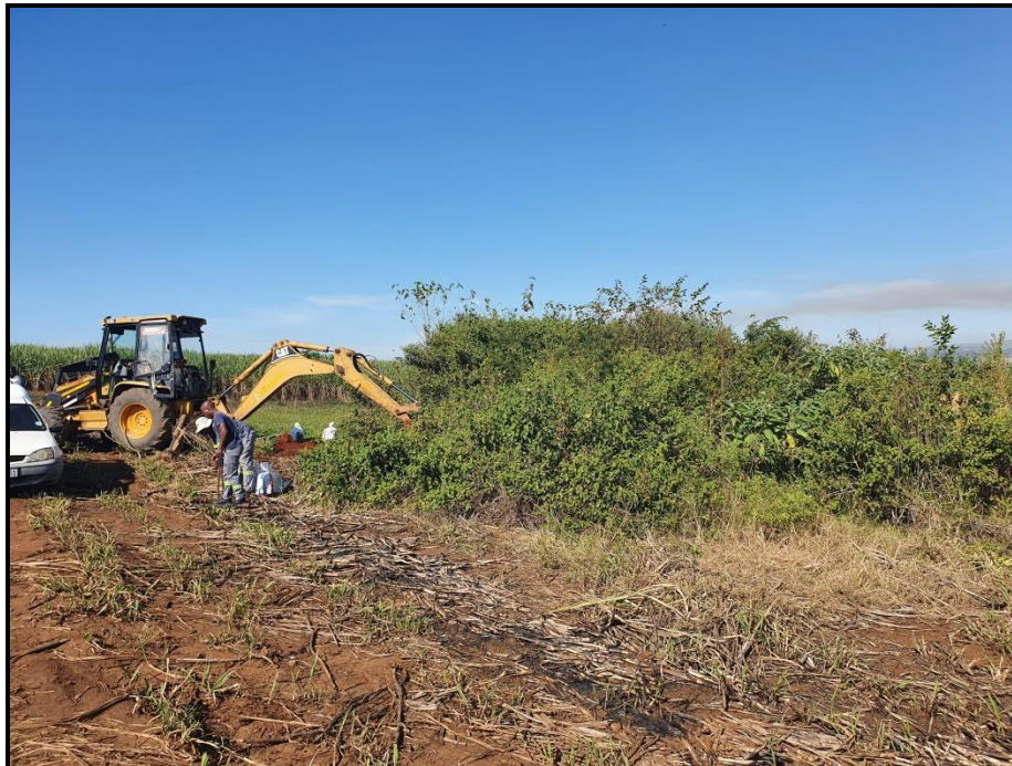
Plate 6: General view of terrain at proposed 1ML reservoir site
