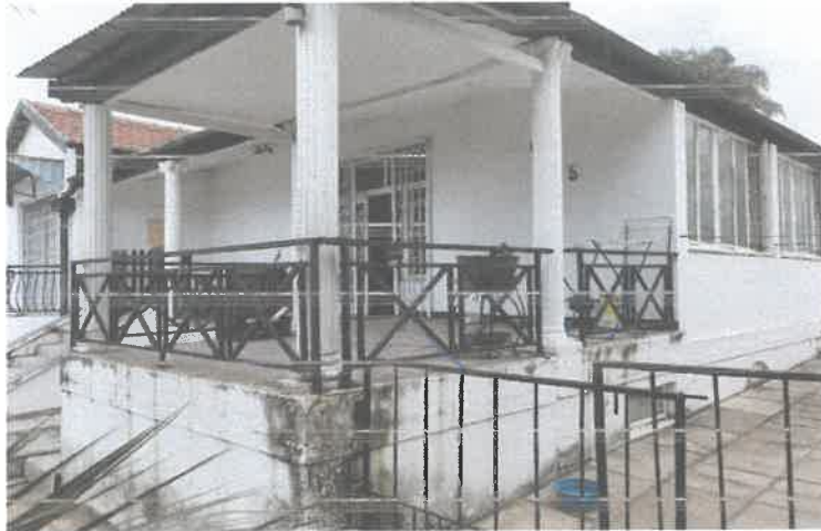
Existing building (Figure 2.5)
