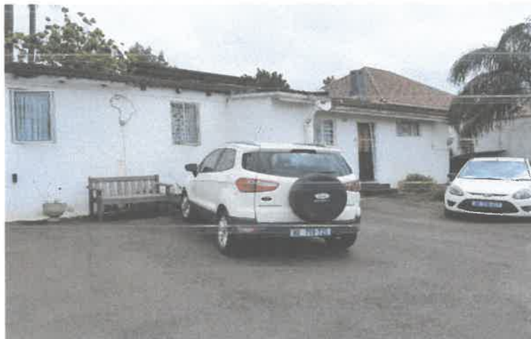
Existing building (Figure 2.7)
