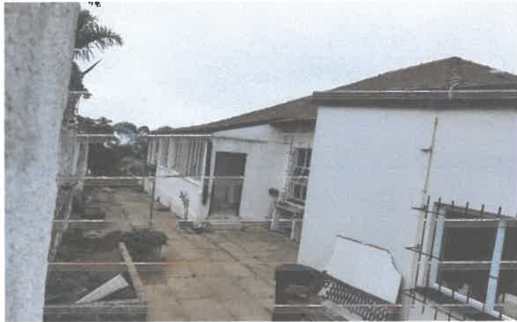
Existing building (Figure 2.6)
