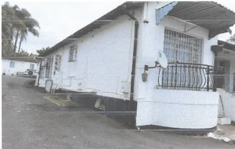
Existing building (Figure 2.3)
