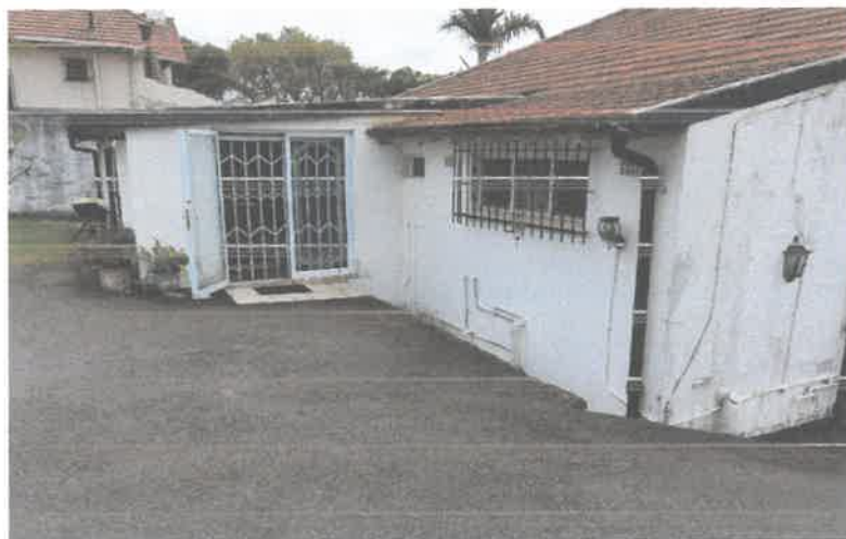
Existing building (Figure 2.4)
