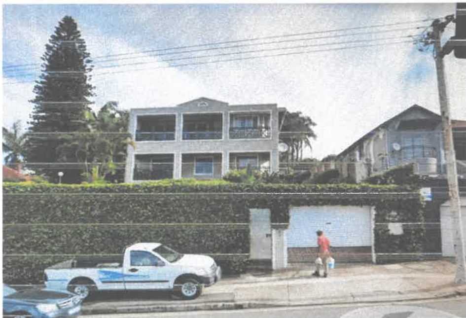
Precedent Building (Figure 2.1)
