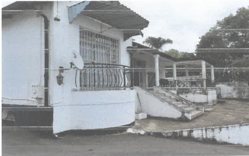
Existing building (Figure 2.2)
