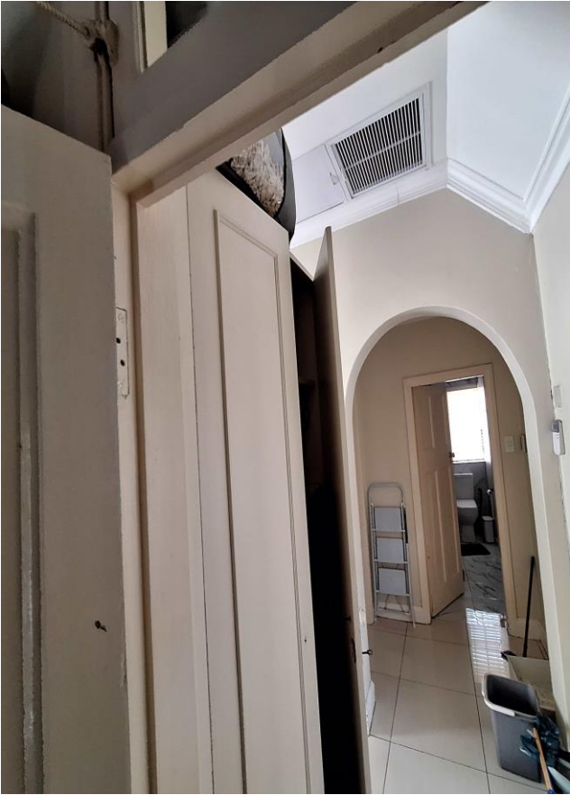
UPSTAIRS PASSAGE LOOKING WEST
