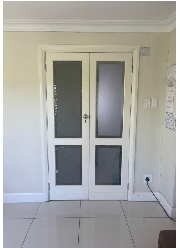
DOORS TO MAIN BEDROOM
