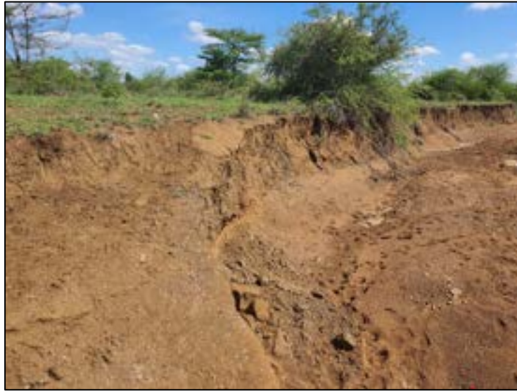
Figure 3-13: View of a large drainage line in Deviation 3.
