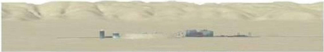
View from 5 000 metres
